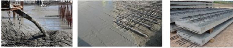
**Reinforced concrete (RC)** is a composite material in which concrete's relatively low tensile strength and ductility are counteracted by adding reinforcement that has a higher tensile strength or ductility.
